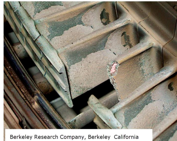
Berkeley Research Company, Berkeley California
