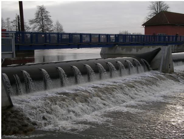
Figure 3: Water filled inflatable dam near Marklendorf
